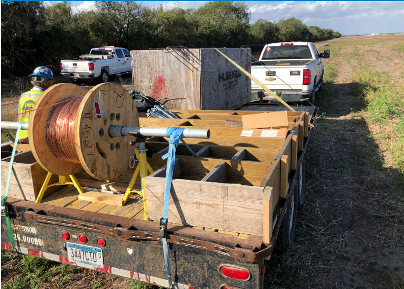
Flatbed trailer organization on a Power Delivery project.
